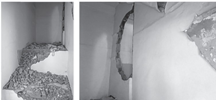
Ilustração 12 - Trace of integration of part of the staircase in the housing space (A wall divided the bearing in two and stairs were processed as two half-levels)
