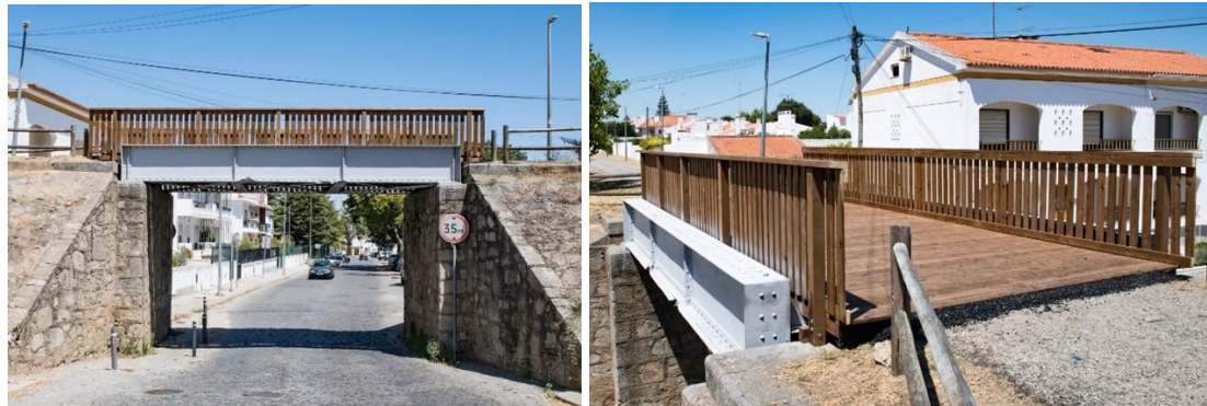
Figures 7 and 8 – Évora Iron Bridge (2022)
