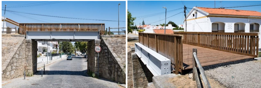
Figures 7 and 8 – Évora Iron Bridge (2022)
